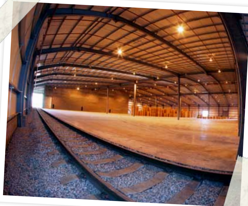
Inside the existing facility
