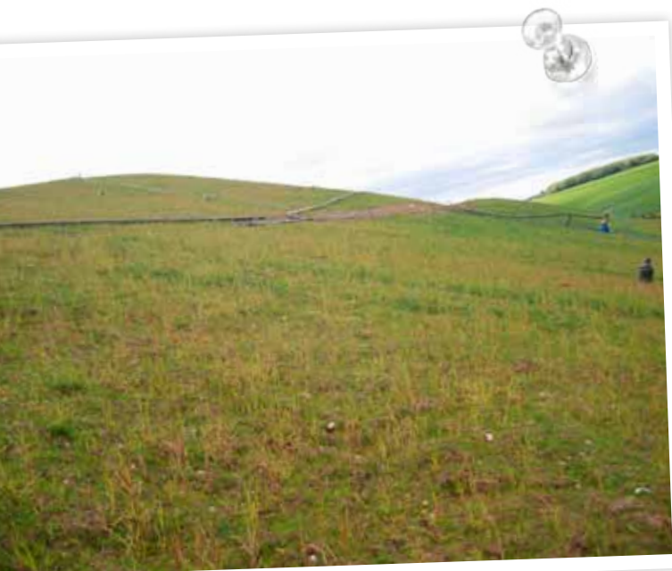
Capped and restored area at Stoneyhill landfill
